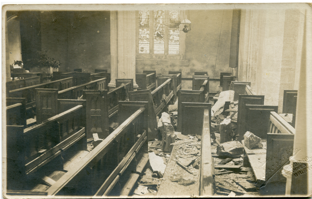
Here we see the interior of the nave in the foreground, with the south aisle behind. Masonry fallen from the top of the tower is strewn among fragments of ceiling plaster and wooden panels from the roof. Some of the pews are standing at odd angles but they have survived well - a testament to their sturdy construction.
