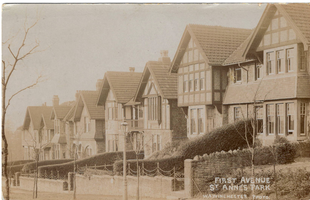
Titled 'FIRST AVENUE ST' ANNE'S PARK', this shows the same short row of houses as in the picture above, but looking downhill. Some of the trees lining the street are still staked, and none have yet been subjected to the pruning that has become so noticeable. Earliest known picture: posted before 3 June 1918 (when the postal rate increased from a halfpenny to a penny).
