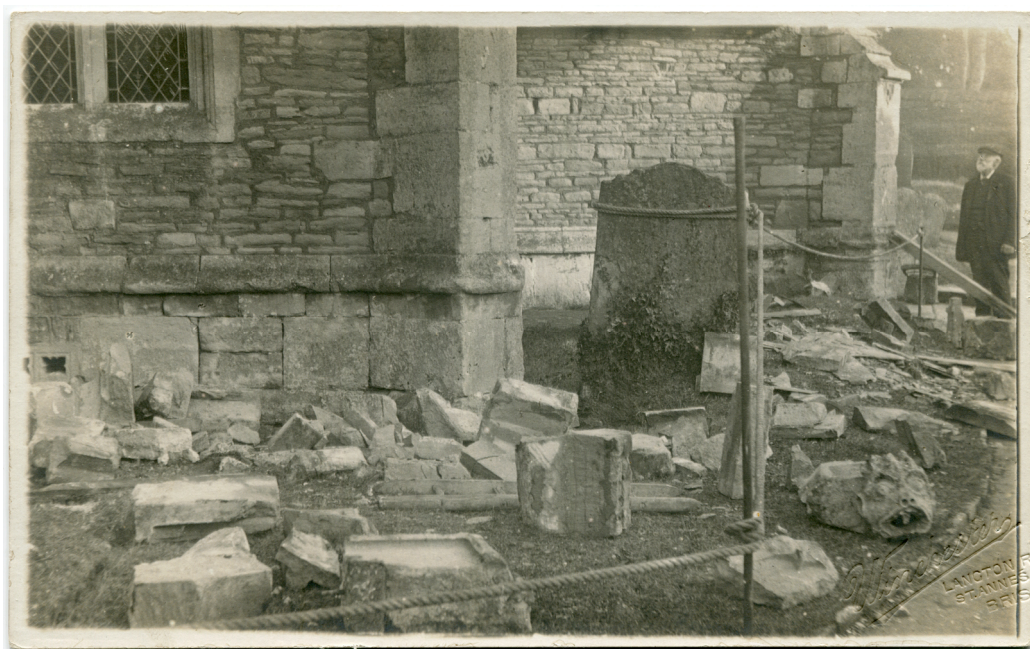
In this photograph we see the fallen masonry has been laid out in the churchyard beneath the tower. The window to our left is at the end of the south aisle (undamaged, and probably the oldest stained glass in the church), and the south porch is to our right. Note the gargoyle in the lower right-hand corner of the picture (enlarged on page 14).
